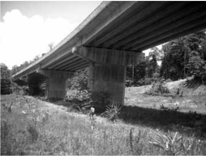
Figure 6. A wildlife viaduct constructed to mitigate the fragmentation effect of highway development in forested areas. The viaduct is designed to allow wildlife to disperse safely between forested areas on both sides of the highway and reduce the number of serious traffic accidents.
